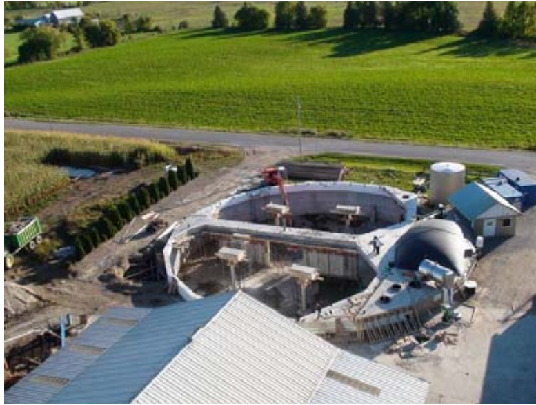
Fig. 4: Fepro Farms Larger Digester under Construction
