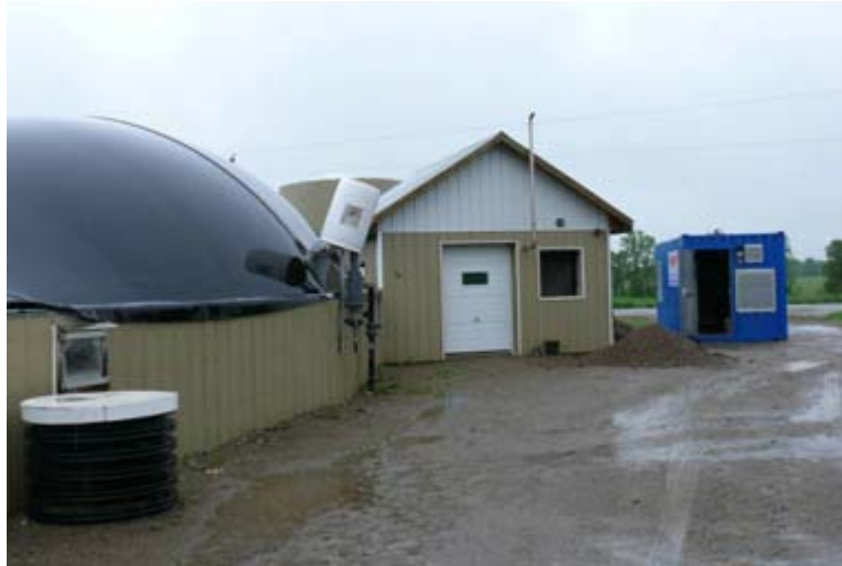
Fig. 1: Picture of Initial Fepro Farms Digester
